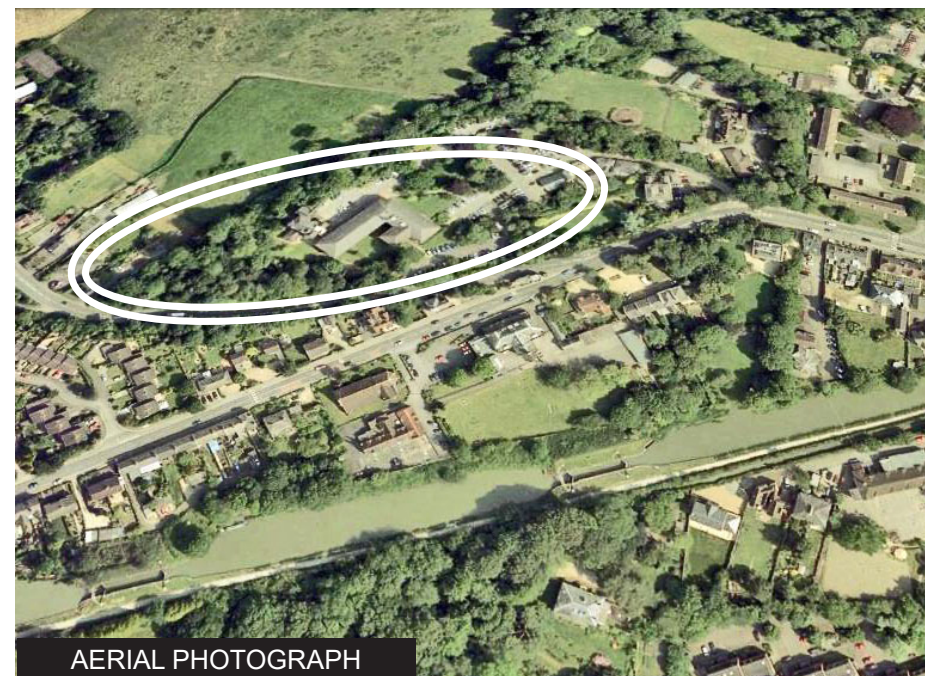
Recent aerial photograph with the general site area site ringed in white.
