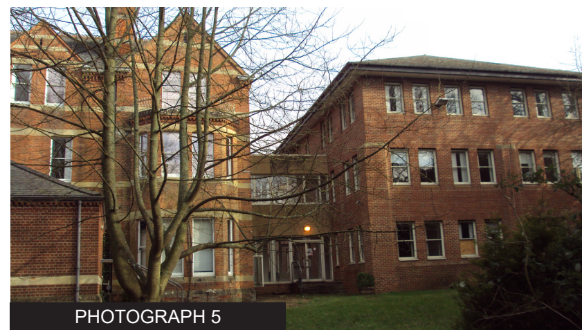
Rear (west) elevation showing link block between original 'Browfort' on LH side and modern office block to RH side
