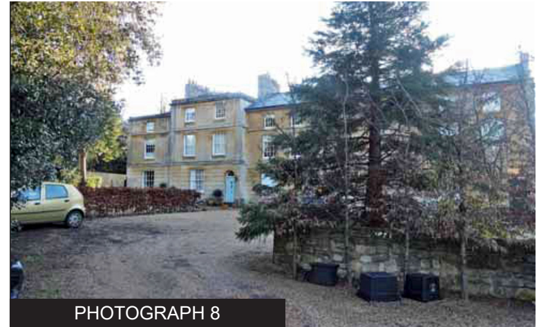
PHOTOGRAPH 8 Trafalgar Terrace - 1-5 Bath Road
